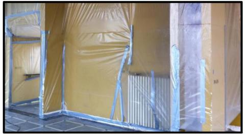
The asbestos removal activity is regulated and sensitive due to the dangerous nature of this product. Therefore, to protect people from these risks, Polyane<sup>®</sup> has developed its unique asbestos removal range: SP ASBESTOS. These white or transparent films bring total security to the work.
